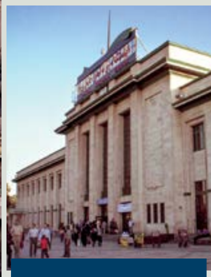
Railway of the Islamic Republic of Iran-Tehran Station
