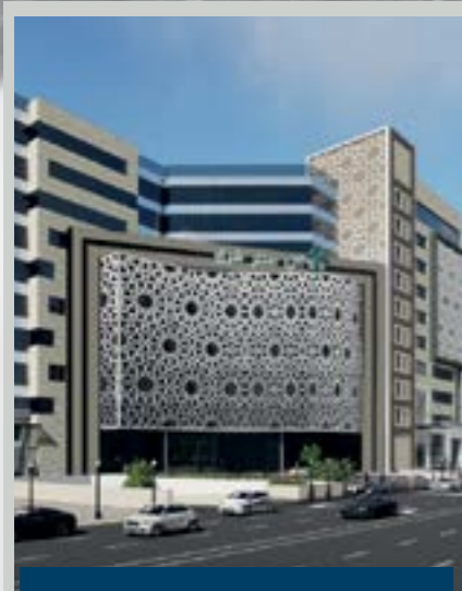
Ati Center Commercial Complex, Mashhad
